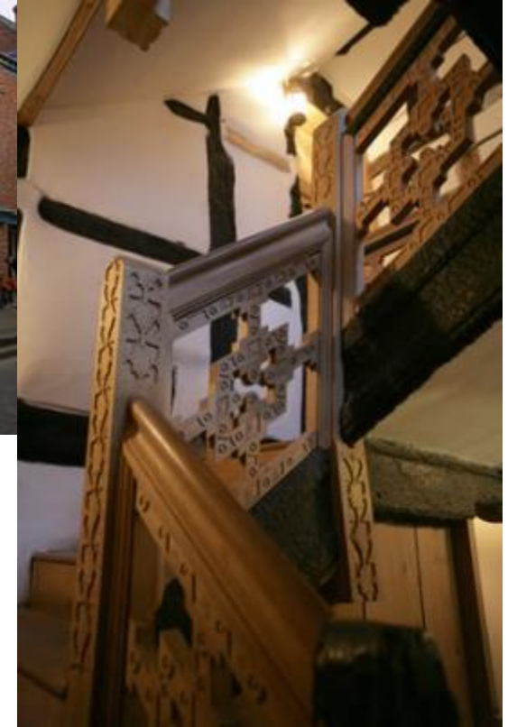
Staircase House, Stockport Rare Jacobean Cage Newel timber staircase
