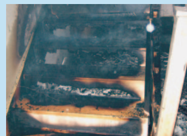
Unprotected stair after test
