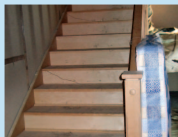
Stair prior to test
